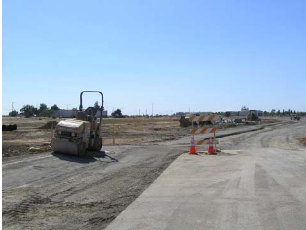
Figure 6. View of project site looking north from CMD Court
