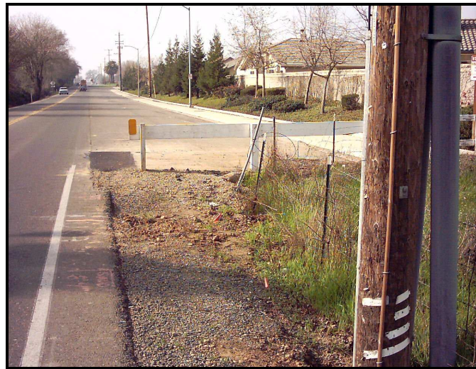
So-called "zipper streets" that combine narrow and wide sections are the result of deferred roadway construction policies in place prior to the incorporation of Elk Grove
